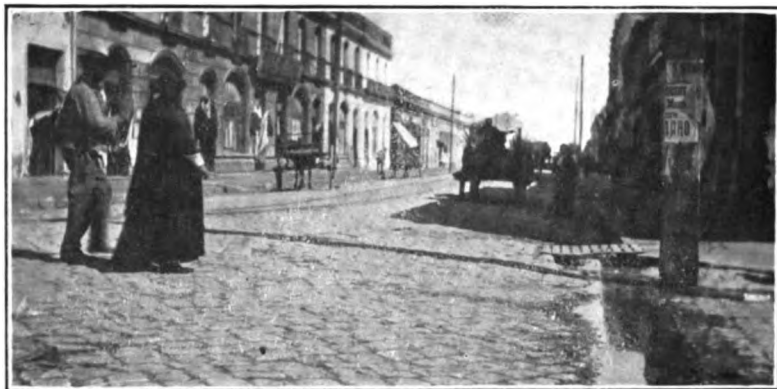
Calle Roble, Chillán, Looking East from Calle Arauco
